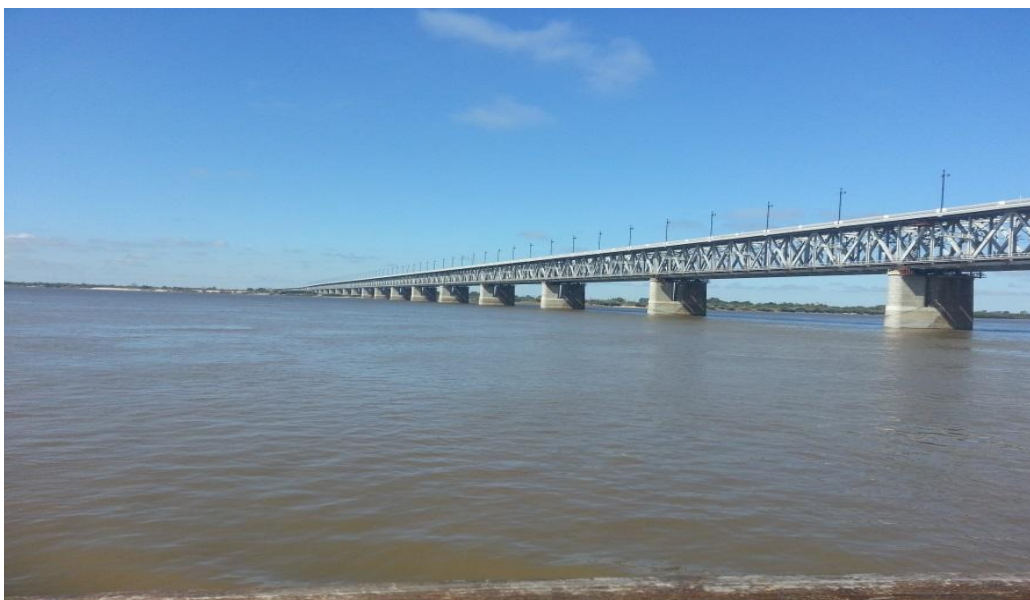
The Transsibirskaya Railroad bridge is most likely responsible for a 0.5–0.7 meter rise in the maximum flood levels near Khabarovsk by Rivers without Boundaries Coalition
