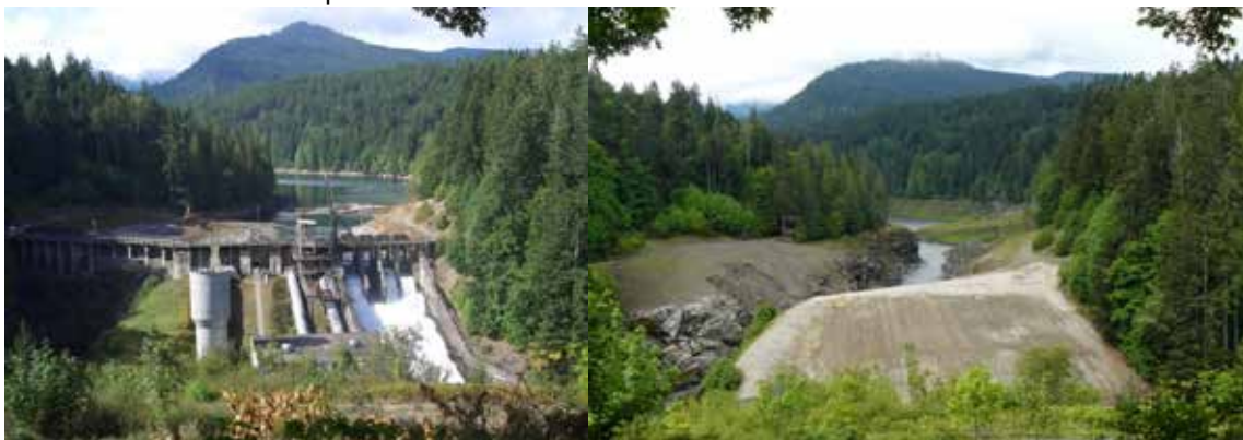
Left: Elwha Dam under deconstruction (Ben Cody/Wikimendia), Right: Elwha Dam Finished, May 2013 ( Zandcee/ Wikimendia)
