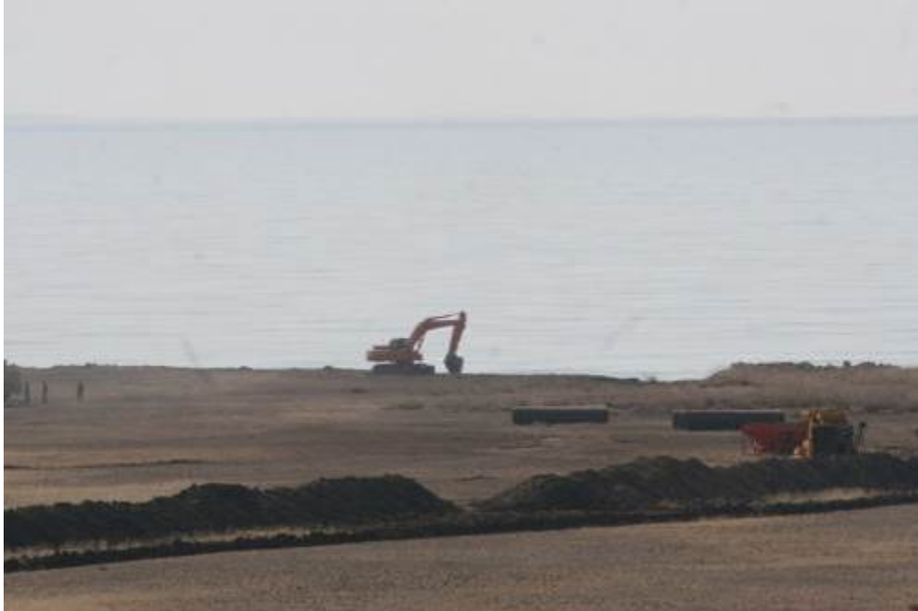
Pipeline construction. Hulunbuir, Inner Mongolia (RwB archives)
