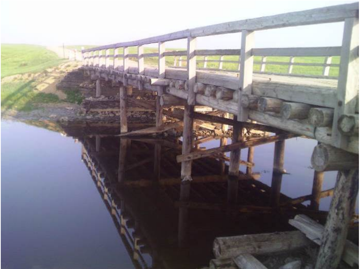
A bridge across a river in Dauria, Tsagan -Ovoo,2013
