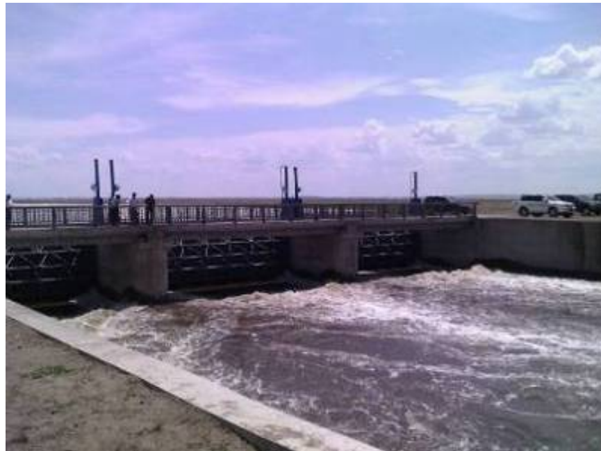
Water intake structure at Hailaer River. 2011
