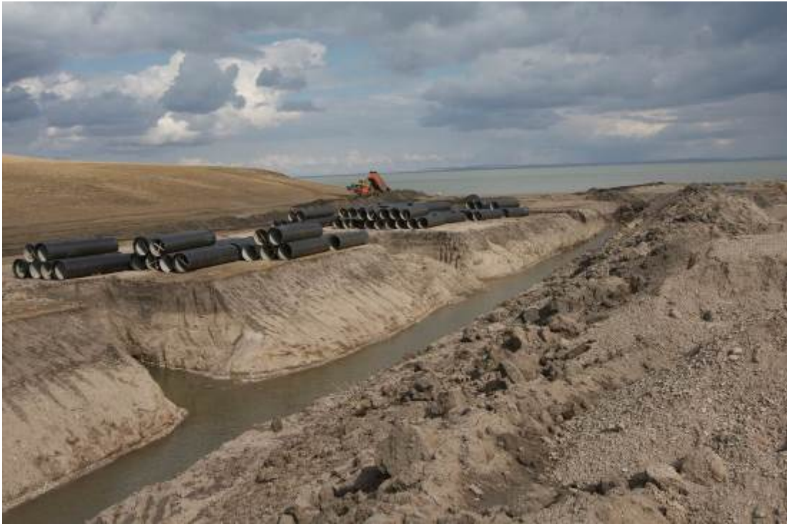
Pipeline construction at Dalai Lake in 2008. Hulunbuir, Inner Mongolia (RwB archives)
