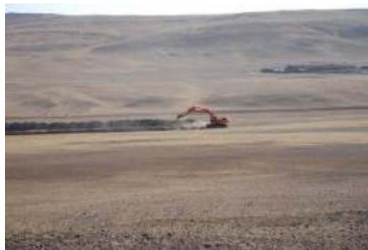
Pipeline construction. Hulunbuir, Inner Mongolia (RwB archives)
